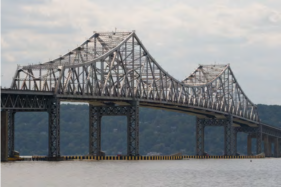
Tappan Zee Bridge clearance 138 feet, elevation mid span 293 ft. (top of spires)
