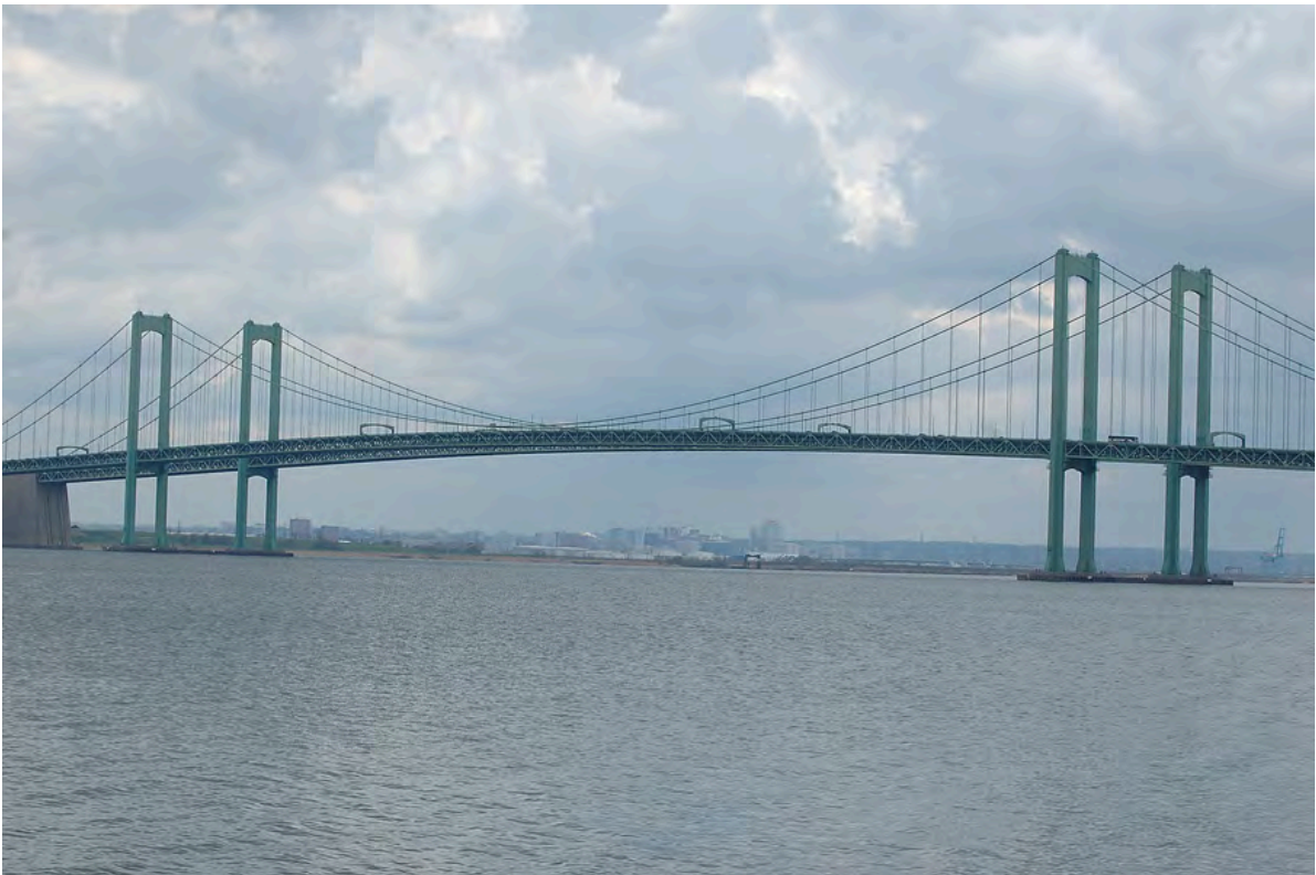
Delaware Memorial Bridge clearance at midspan is 175 ft. and tower height 440 ft.
